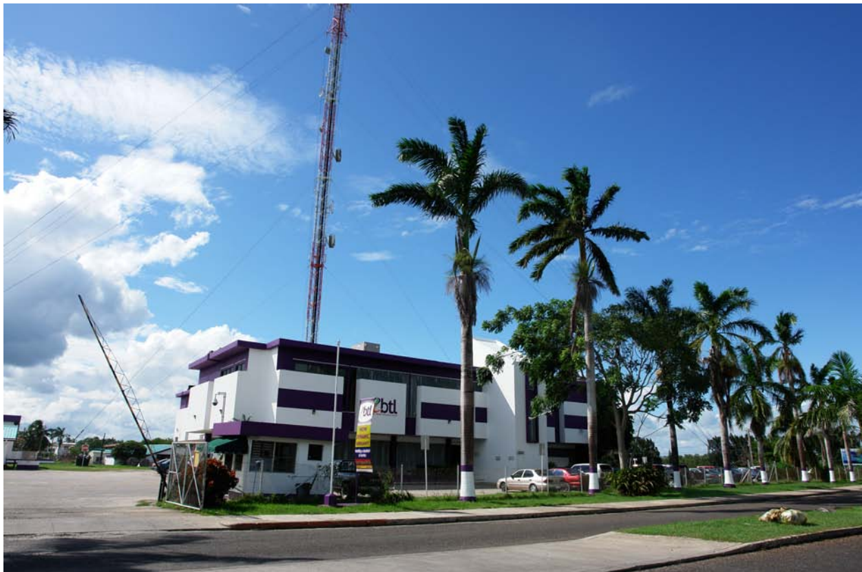
Esquivel Telecom Center, Corporate Headquarters
